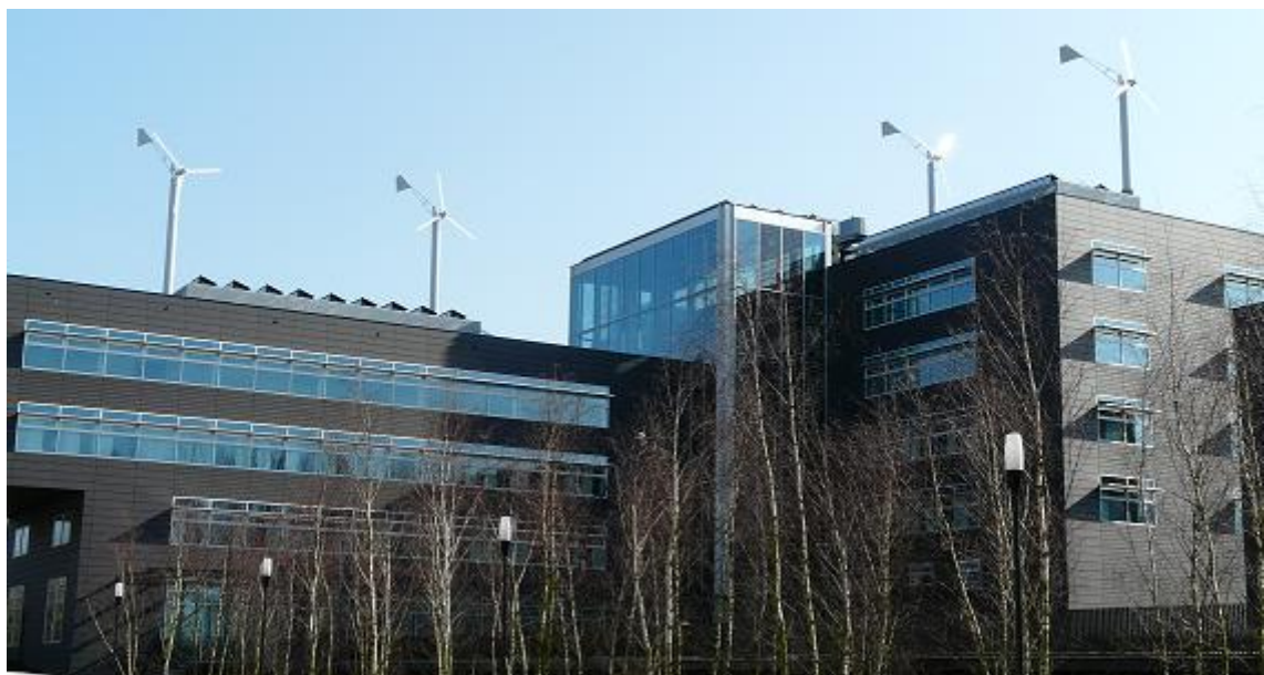
Application: 4 units of Montana on Rabobank The Netherlands
