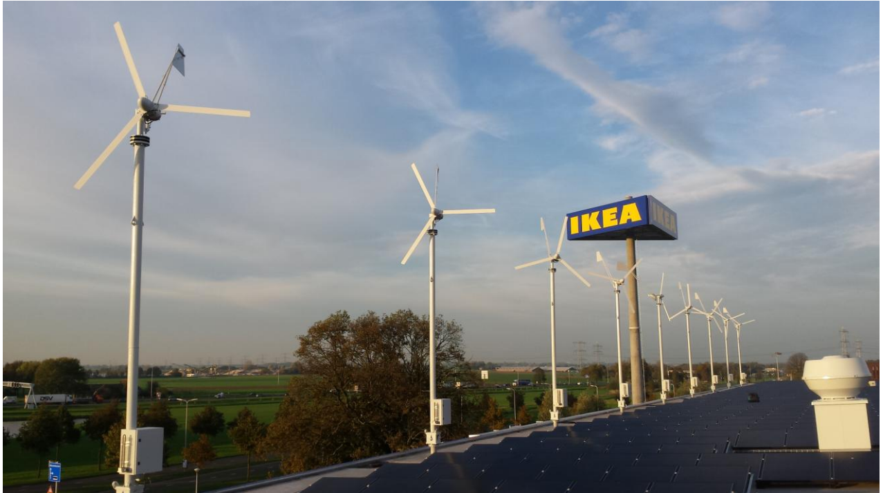
Ikea store in Zwolle, The Netherlands with 9 units of Passaat 1.4 kW
