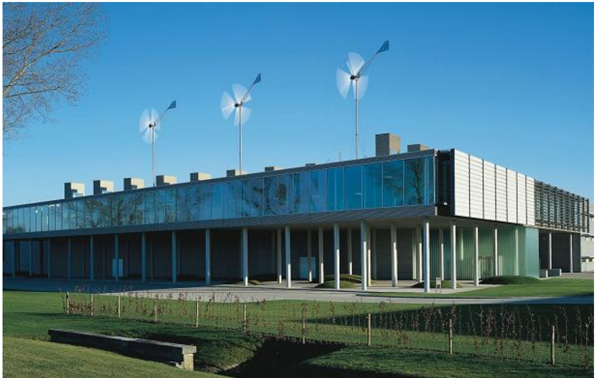
Application: 3 units of Montana on guyed tower in Belgium
