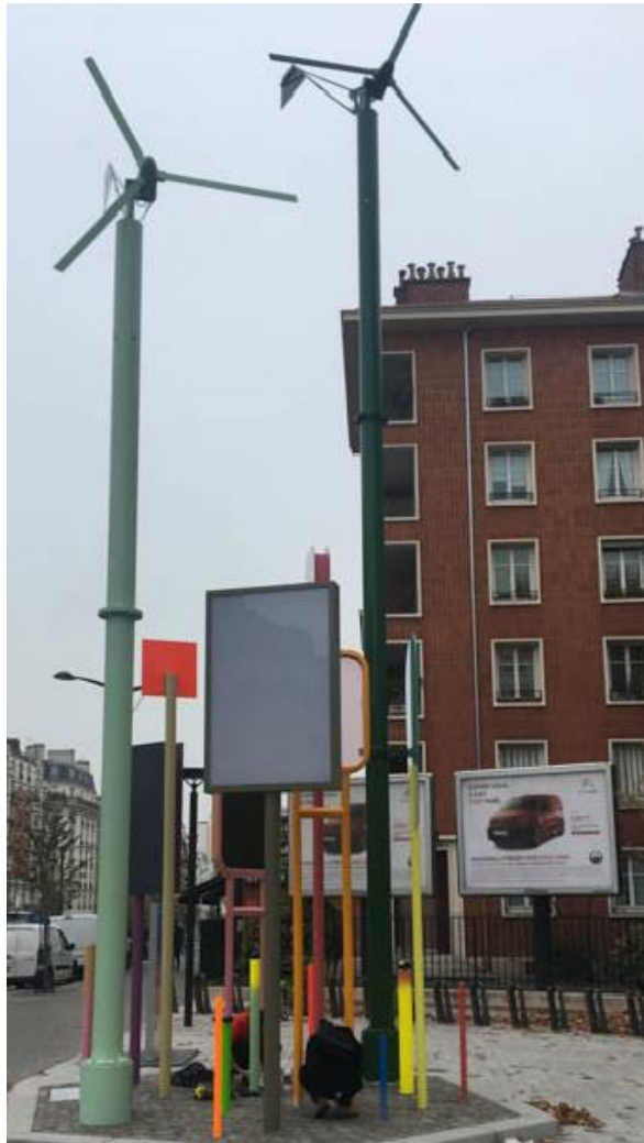
Two Passaat wind turbines energizing signage boards on the left side
