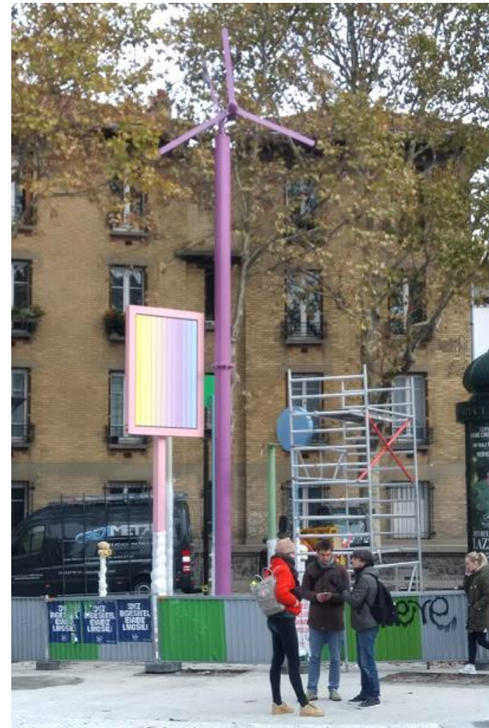
One Passaat wind turbine energizing a LED lightning panel on the right side
